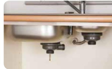
2. Before installing your undersink trap we recommend lining your trap up to all sink connections to make sure you have enough adjustability within the trap and to make sure the outlet of your trap can be connected to your waste pipe. It's at this stage where if required you should shorten any of the adjustable lengths.
