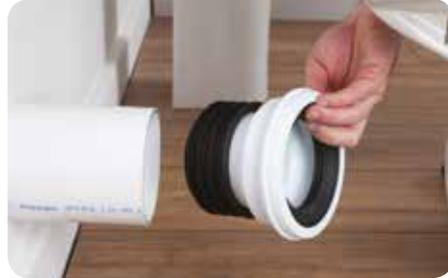
2. Place the finned section of the pan connector into the soil pipe. Depending on the installation it may be more suitable to install the pan connector on the toilet first.
