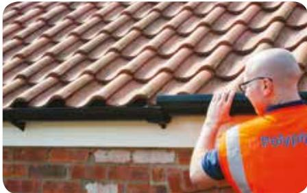
3. When installing your gutter into a run of fascia brackets you should start by connecting the back edge of the gutter under each bracket as demonstrated in this installation.
