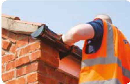
5. Connecting to fittings is the same process as in point 4. Prior to connecting your gutter you will need to make sure it does not go beyond the expansion line, which is detailed on each fitting.
