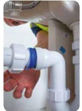
5. When connecting your trap to your waste pipe it's important that the waste can be fully inserted into the outlet of the trap. Once this has been done you can then move the blue finned seal along the waste pipe into the trap.
