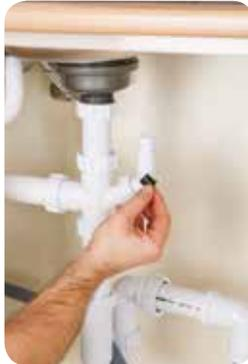
9. Once the cap is removed or the hose end has been cut away, you can connect your hose to the hose connection. Place the appliance hose as far over the hose connection as is possible making sure there are no kinks in the hose once it has rested.
