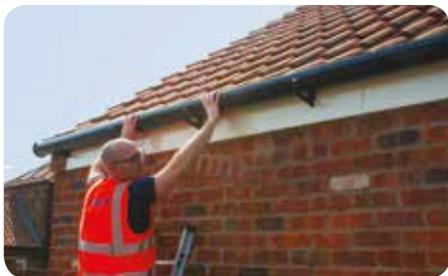
4. Once the back edge of the gutter is in place, the front edge can be clicked into place. It's best to have your gutter in the correct position prior to connecting the front edge as it can be difficult to move the gutter along the run of fascia brackets once it's in place.
