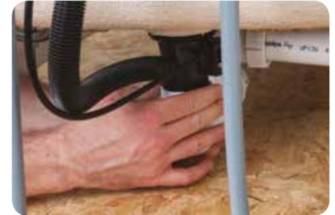
9. Once the installation is complete run water through the trap and waste system to confirm the trap has been installed correctly.
