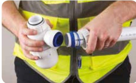
3. When connecting your trap to your waste pipe It's important that the waste can be fully inserted into the outlet of the trap. Once this has been done you can then move the blue finned seal along the waste pipe into the trap.
