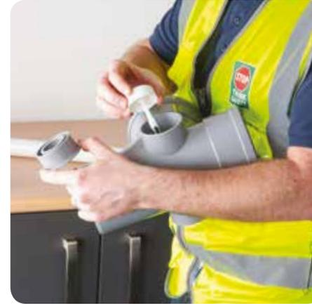
5. Also apply solvent cement to the entire outer surface of the boss adaptor.
