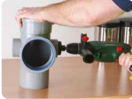
3. Once drilled, remove any loose plastic and de-burr all edges. Apply solvent cleaner to inside surface area of the Boss connection prior to applying solvent cement.
