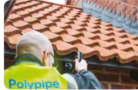
2. Depending on the age and type of roof, the distance between rafters can vary, but on most properties the distance should be around 600mm. We recommend installing a fascia bracket on every rafter.
