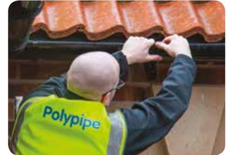
5. Connecting to fittings is the same process as in point 4. Prior to connecting your gutter you will need to make sure it does not go beyond the expansion line, which is detailed on each fitting.
