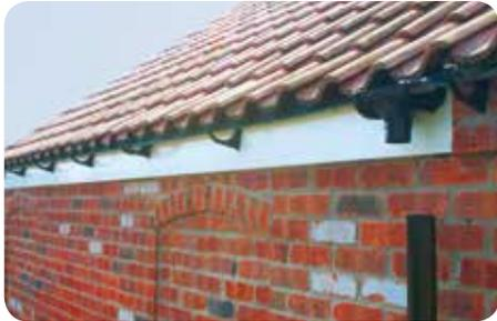
2. Polypipe union brackets and running outlets can be used in place of fascia brackets when the installation allows.
