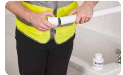
5. The spigot should be inserted into the socket immediately, with a slight twisting action.
