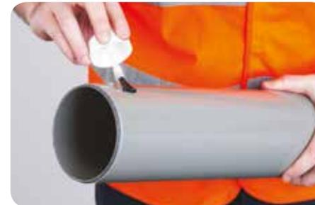
3. Use Polypipe cleaning fluid CF250 to remove any surface grease from the spigot and socket to be jointed.
