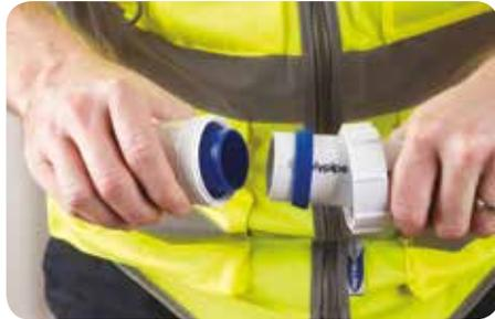
5. Insert the pipe into the fitting.
