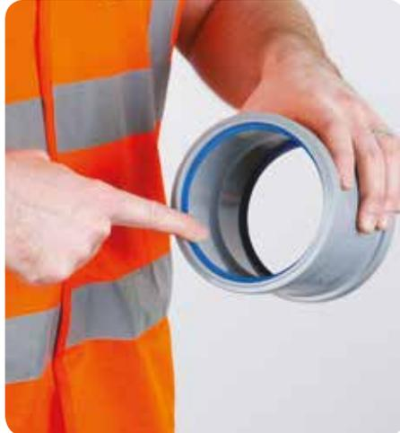
4. Insert the pipe or fitting into the socket and then withdraw it by approximately 10mm to allow for expansion of the pipework.
