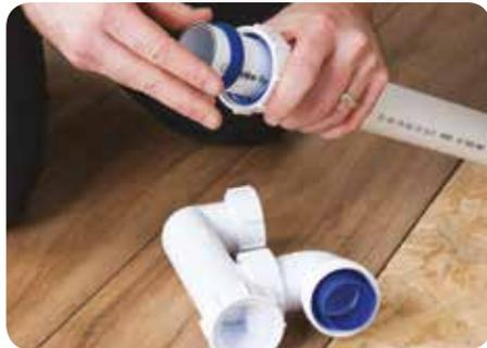
4. When connecting your bath trap to your waste pipe it's important that the waste can be fully inserted into the outlet of the trap. Once this has been done you can then move the blue finned seal along the waste pipe into the trap.
