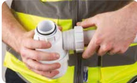
4. Once the seal is in place, the threaded nut can be threaded onto the trap, which will create a compression seal between your waste pipe and trap. After the threaded nut has been hand tightened a final ¼ turn is required. A final inspection of the connection is required to make sure the connection has been made by pulling on the pipe and fitting. This may not be suitable in certain applications.
