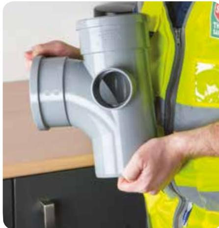
4. Apply solvent cement to the entire surface of the inside of the boss socket on the soil fitting.
