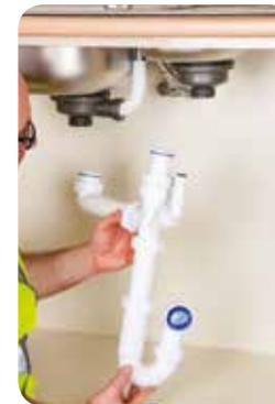
3. When connecting your trap to your sink outlets the seals need to be 100% flush with the outlet. If this is not the case then you may need to use the adaptor provided with your undersink trap along with the seal for this adaptor.
