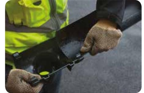
4. When connecting a piece of gutter to a gutter fitting, it's best to start by placing the gutter under the flexible clip which is facing away from you. Once the gutter is positioned under the flexible clip you can then move the front edge of the gutter under the flexible clip closest to you.
